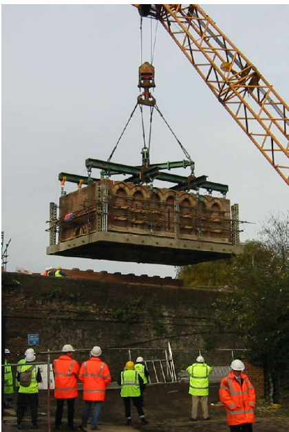
A section of the Waterpoint being lowered into position
