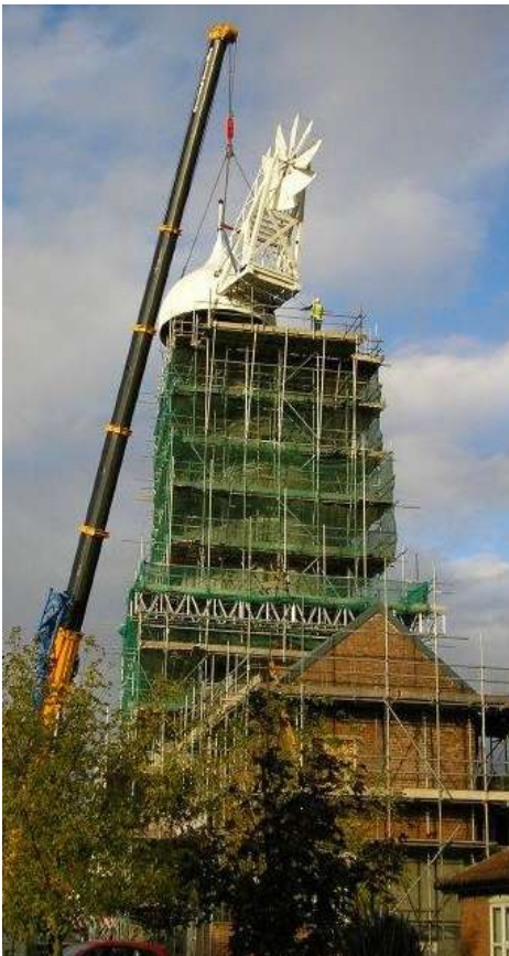
The new mill cap being lowered into position
